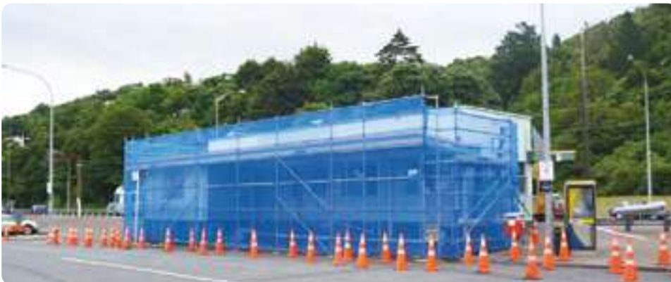
Figure 3: Covered scaffolding on a single storey building.
