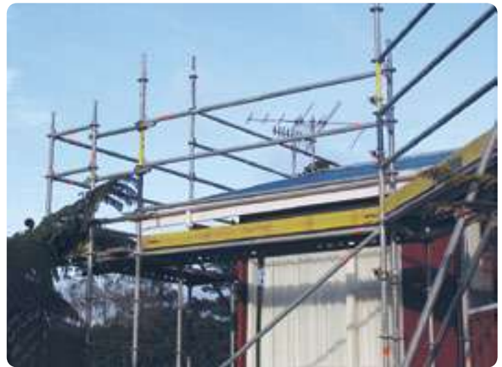
Figure 7: Example of edge protection on a roof of a residential home.
