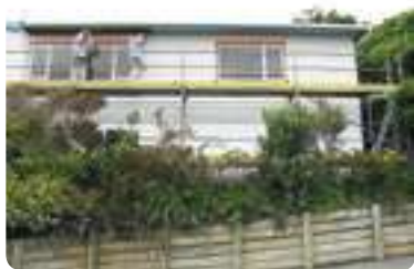
Figure 4: Scaffolding on a residential building.
