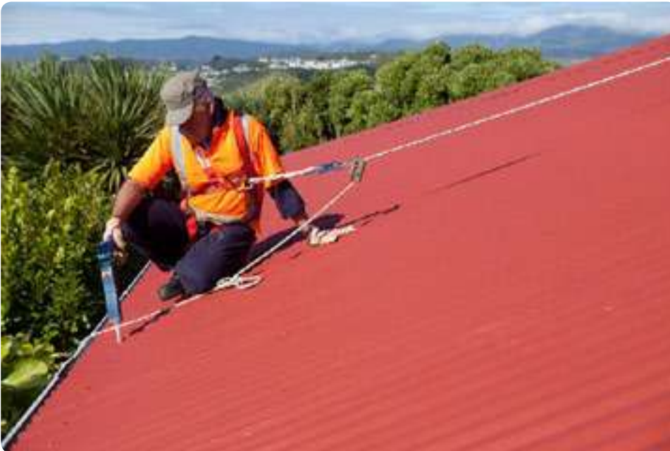
Figure 13: Minor roof repairs can be undertaken with work positioning.
