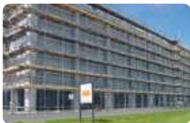
Figure 5: Scaffolding on a multi-storey building.
