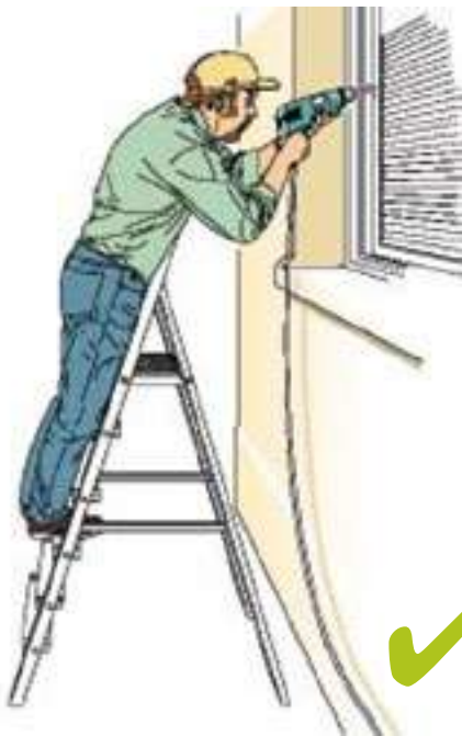
Figure 30: Correct – steps facing work activity.
