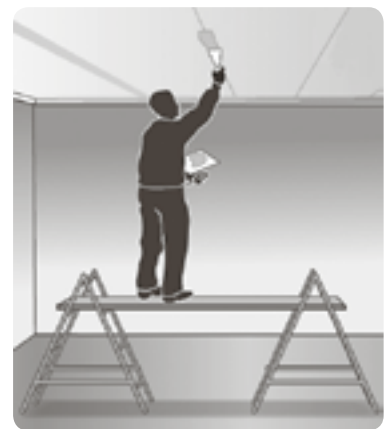
Figure 24: A worker stands on a trestle scaffold.
