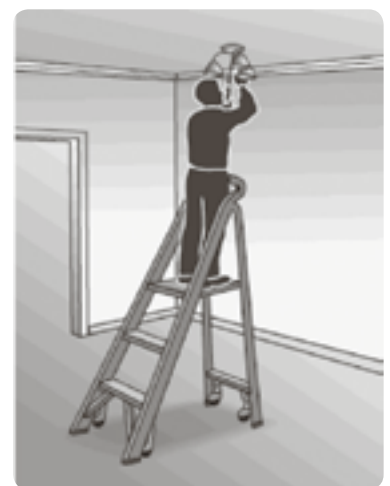
Figure 25: A worker uses a step platform.
